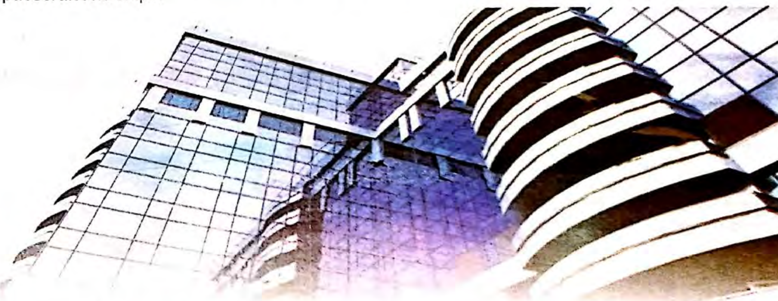
Figure 6.8 Aluminum abundantly use in High-rise buildings
